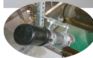
WCM411 sensor installed over a silo feeder belt
